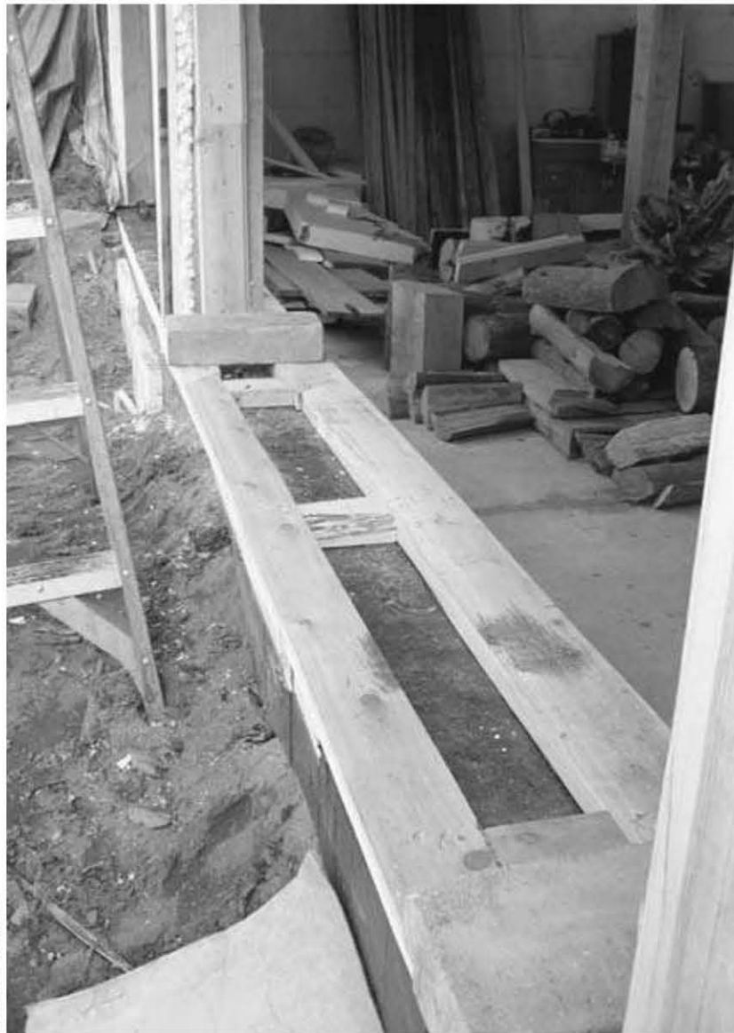
Fig. 12.2: The poured wall is broadened to accommodate the 16-inch cordwood wall by the use of this 2 × 6" detail, described in the text.
