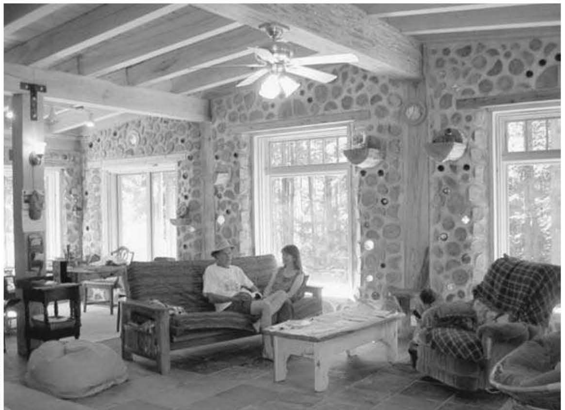
Fig. 12.3: Mark and Mary in their new home. The engineered paralam beam overhead spans 18 feet.
