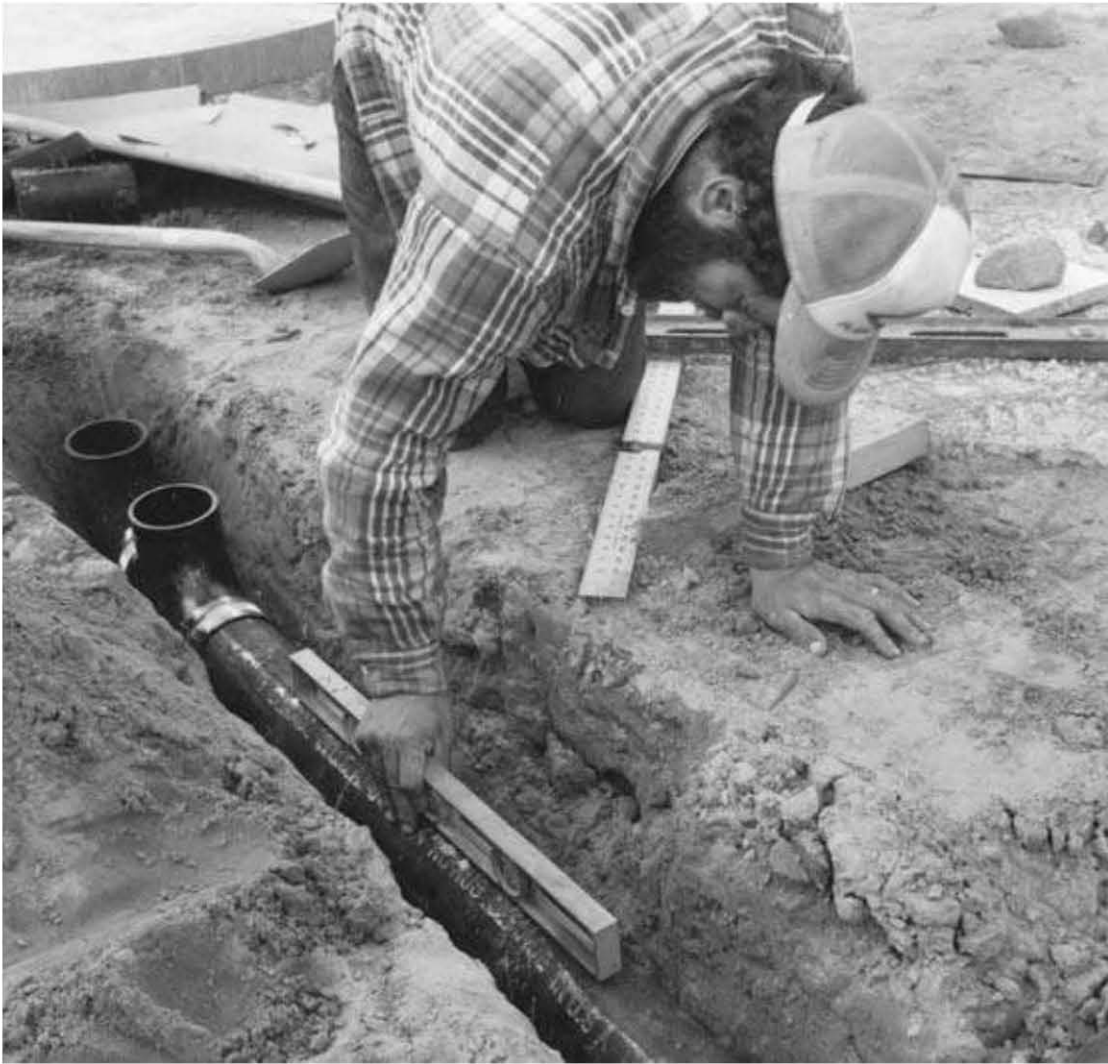
Fig. 4.10: Installation Tips for Underfloor Plumbing Dennis Lee Plan the plumbing so that all traps are accessible. In the case of a bathtub or shower on the first floor, this will usually necessitate “boxing out” a small area so that concrete cannot get in around the trap or drain. An 18-inch square box made of 2-by-6 material can be seen in Figure 4.9. It provides access to our shower drain and trap. Another good reason for the box is that – thanks to the ubiquitous Mr. Murphy of the famous law – it is very difficult to get the drain in exactly the right place with respect to adjacent walls, which are still non-existent at this point in time. Within the box, you can still make final adjustments to a drain location at the time of shower- or tub-base installation.
