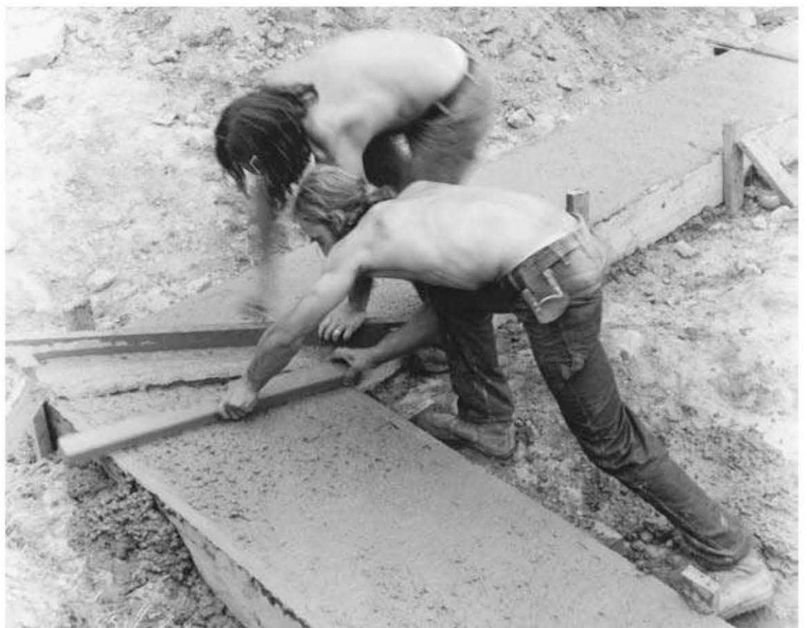
Fig. 3.23: The concrete is screeded with a short, straight-edged board.
