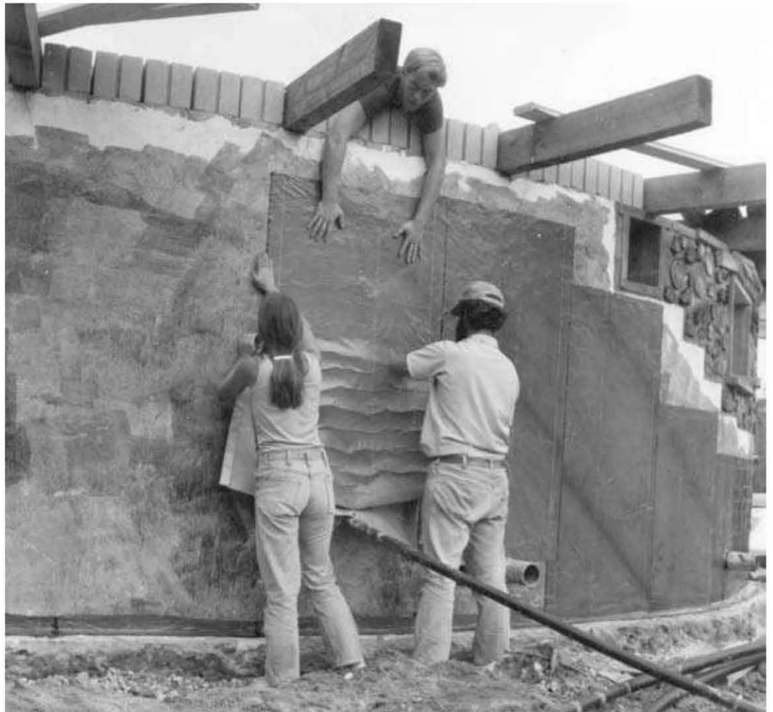
Fig. 7.2: Bituthene ® waterproofing membrane is applied vertically to walls.
