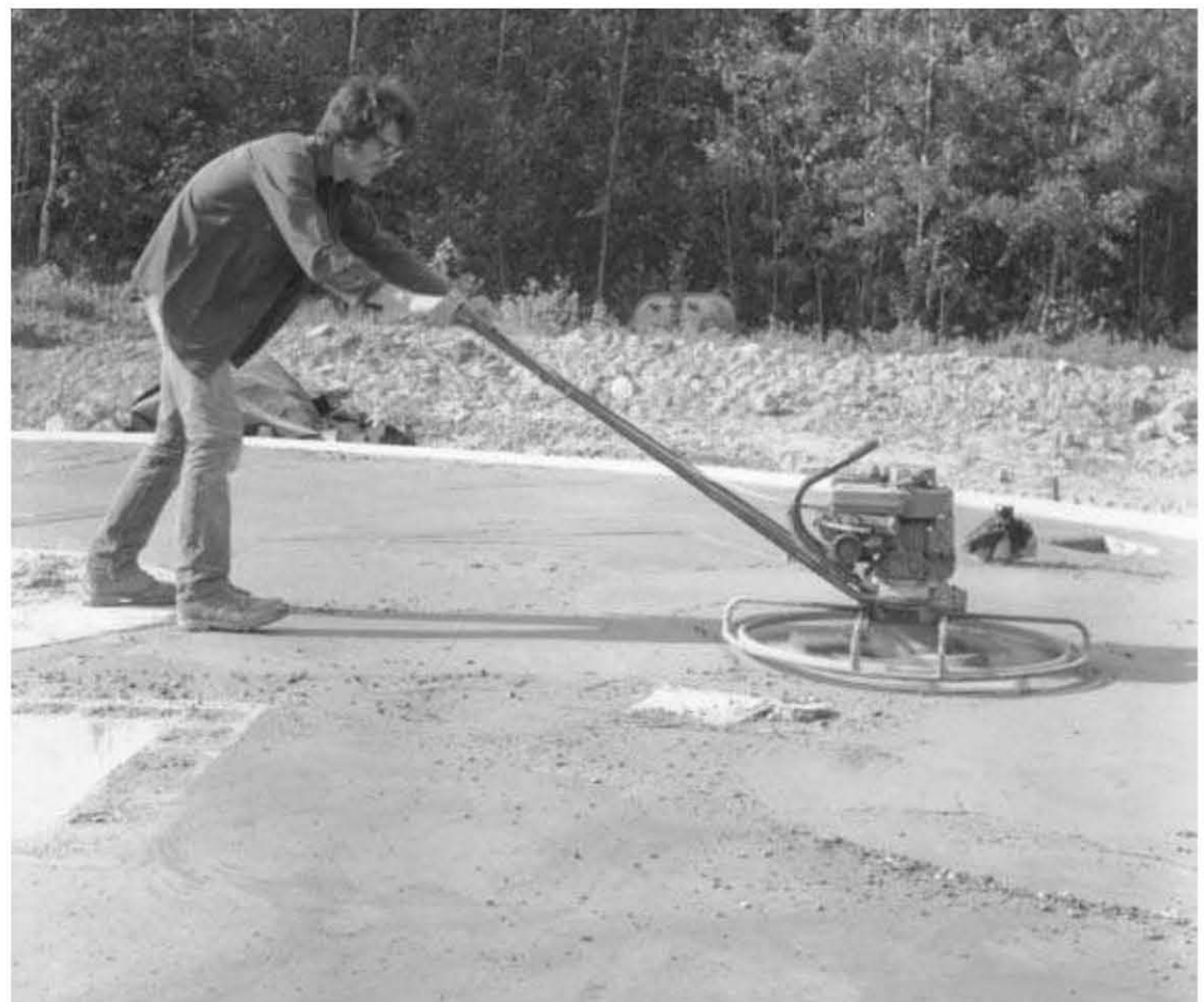
Fig. 4.17: Jonathan Cross power-trowels the slab at Earthwood.
