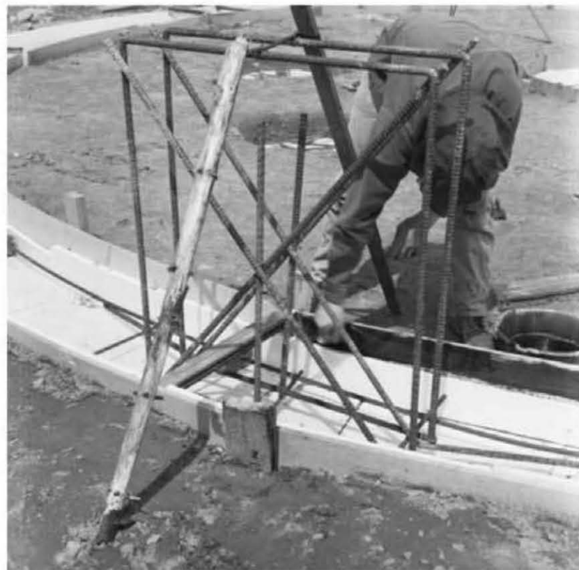
Fig. 3.19: At Earthwood, the buttress cage is made of #6 ( \frac{3}{4} " ) rebar.
