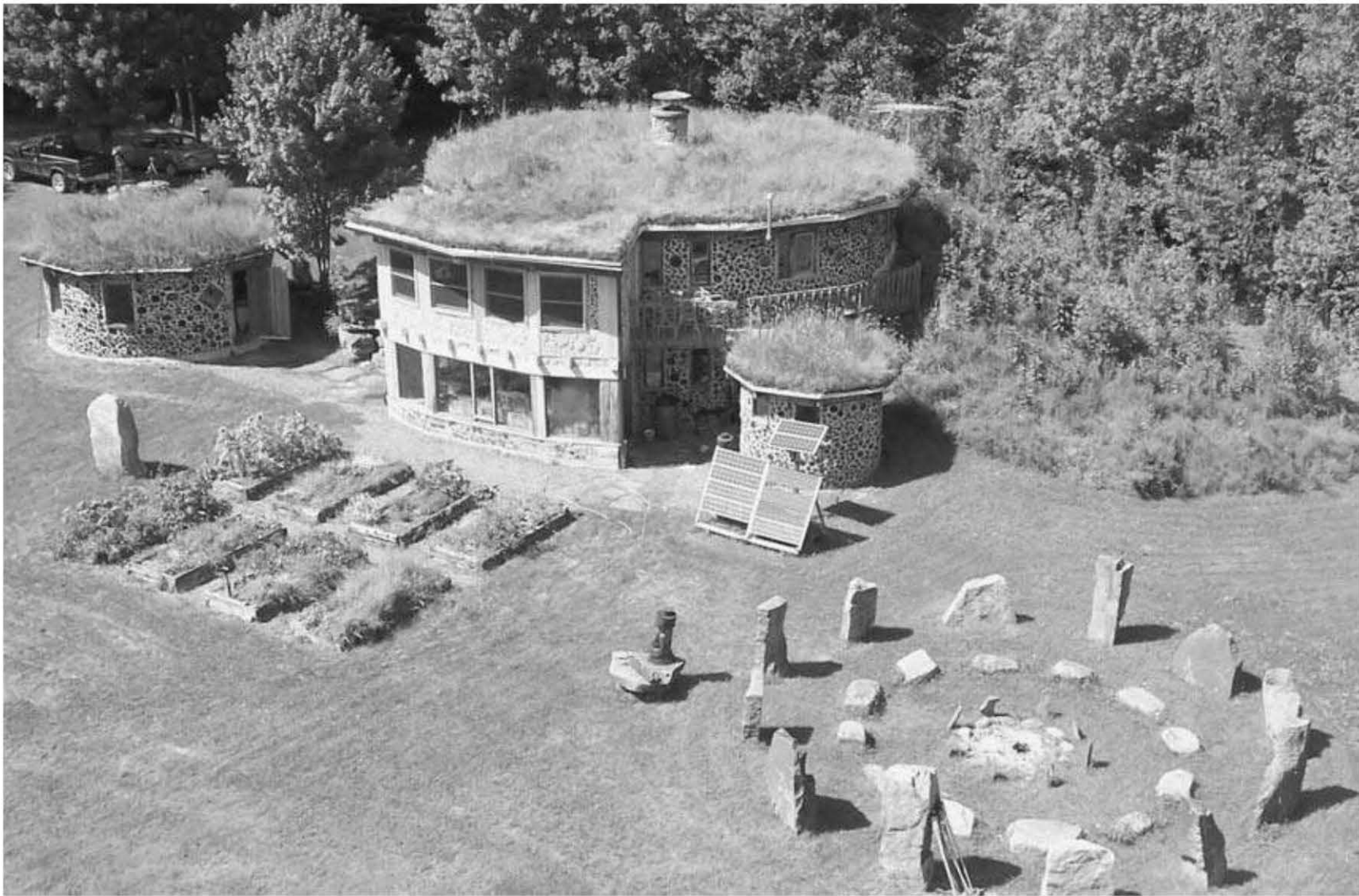
Fig. 9.6: Earthwood, as seen from halfway up the 108' windplant tower.
