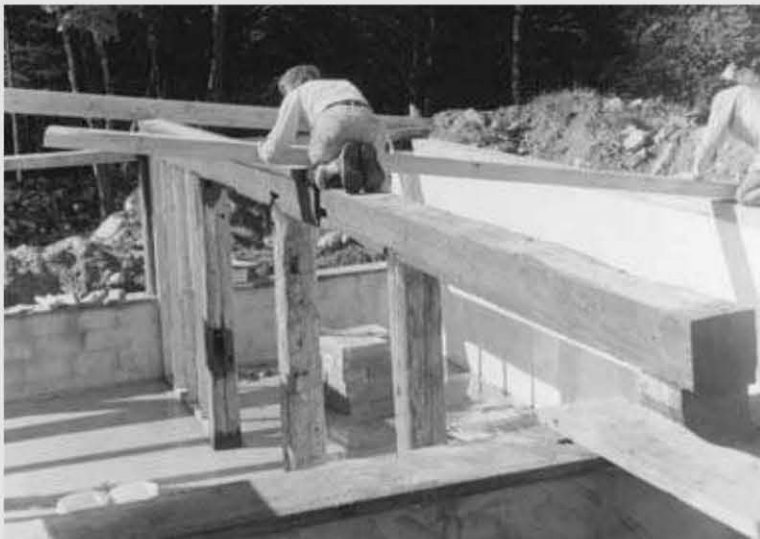
Fig. 6.8: We slide a rafter along the girders.
