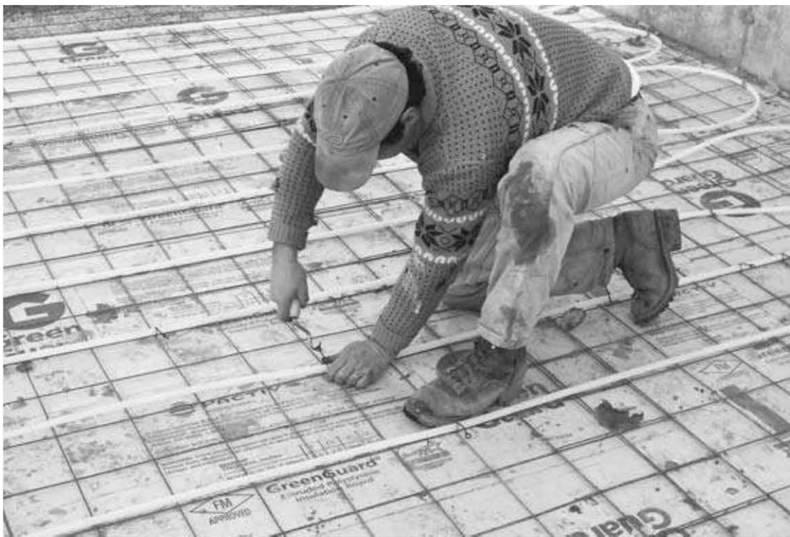
Fig. 4.6: Steve Bedard fastens his polyethylene tubing to the wire mesh with a special rotating hook made for twisting tie bands.
