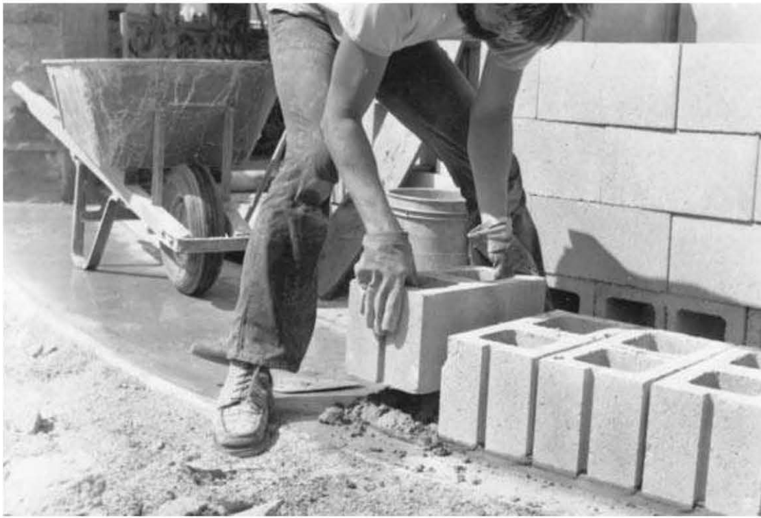
Fig. 5.10: The prudent course of action is to have your wall plans checked by a structural engineer, who can advise you on the need and placement of bond-beam courses and filling cores for bearing pillars. Earthwood: the first course of 8" corner blocks is set in mortar.
