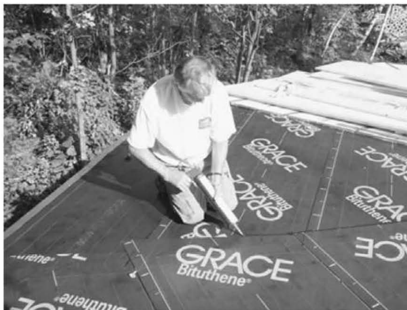
Fig. 8.2 (right): The author caulks the cut edge with Bituthene® Mastic.
