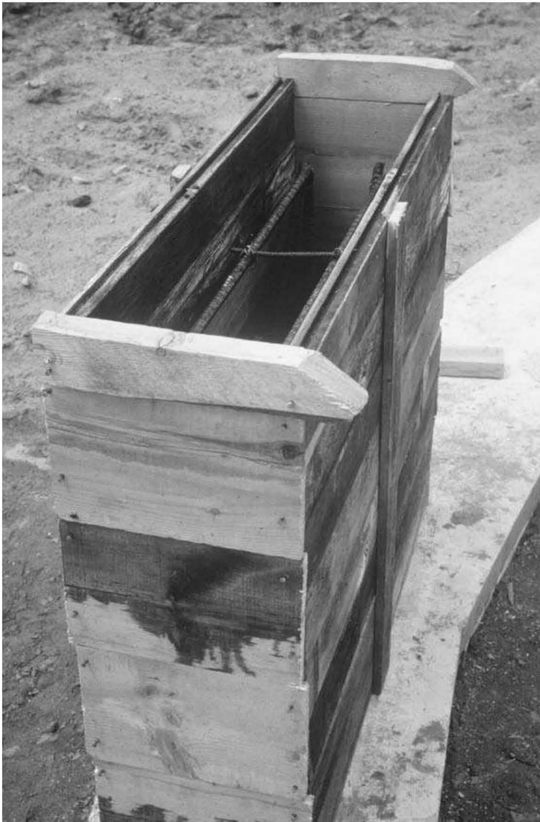
Fig. 4.16: We formed the buttresses with recycled 2 × 6" tongue-and-groove silo boards. of the sand to slow the set. And (3) Specify two trucks, maybe 45 minutes apart, so that there is no waiting for the second half of a large pour.
