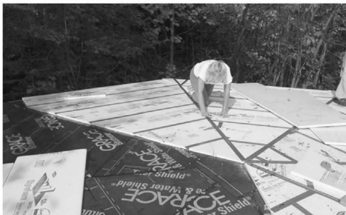
Fig. 8.2 (right): The author caulks the cut edge with Bituthene® Mastic.
