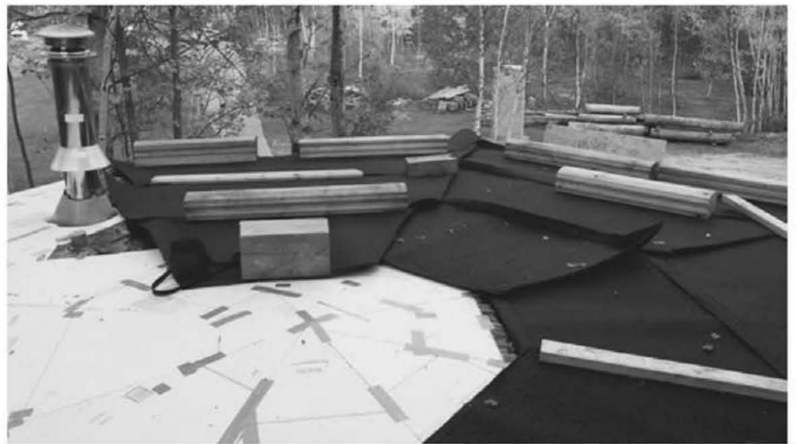
Fig. 8.6 (below): Trapezoidal sheets of Enkadrain® 3615R composite drainage are placed over the plastic, with the filtration mat uppermost. No, we haven't forgotten the plastic sheet. You can see it poking out here and there. A large centerpiece of plastic will be tucked under the Enkadrain® before it is covered with earth. Heavy wooden blocks keep everything in place until the earth goes on.
