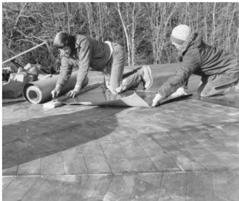
Fig. 7.7: Cut Bituthene® with a razor knife, over a scrap board.
