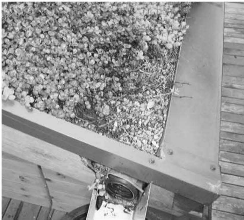
Fig. 8.23: Photograph of the drainage detail at the Dancey home.
