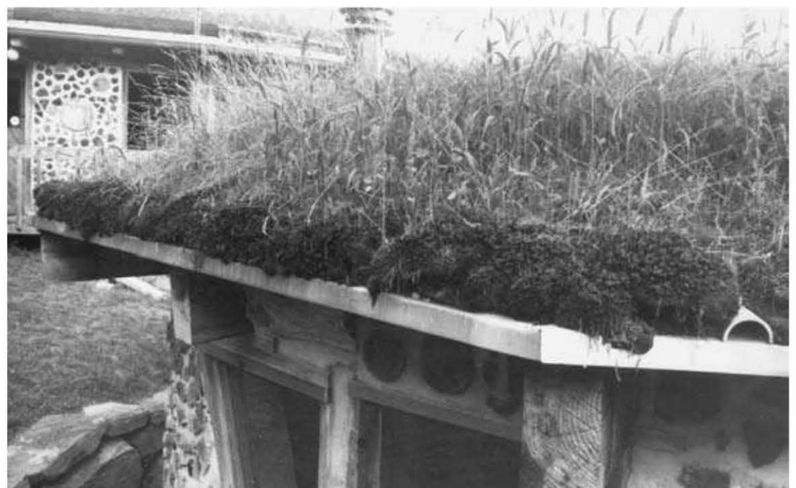
Fig. 8.18: Moss sods drain well, retain the earth and look natural. Note "half-pipe" for drainage.
