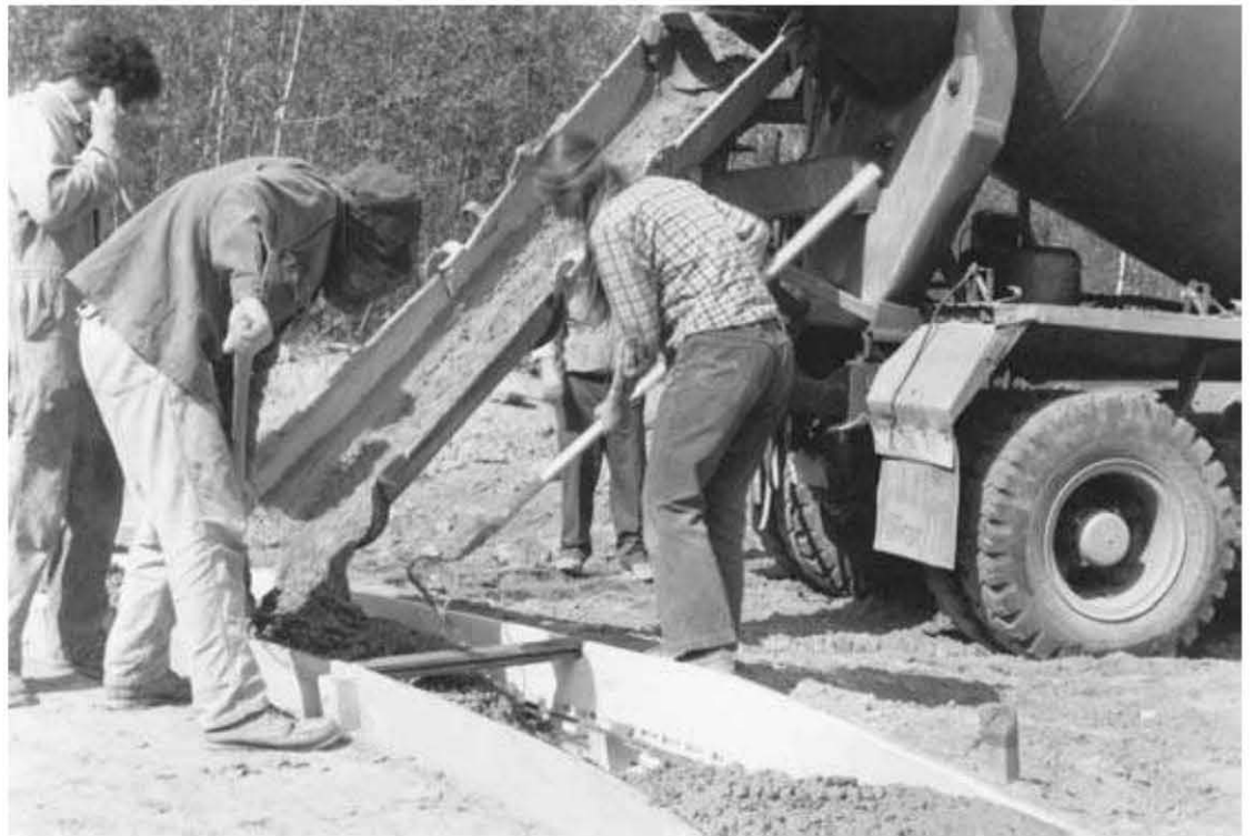
Fig. 3.22: Pouring the footings at Earthwood.
